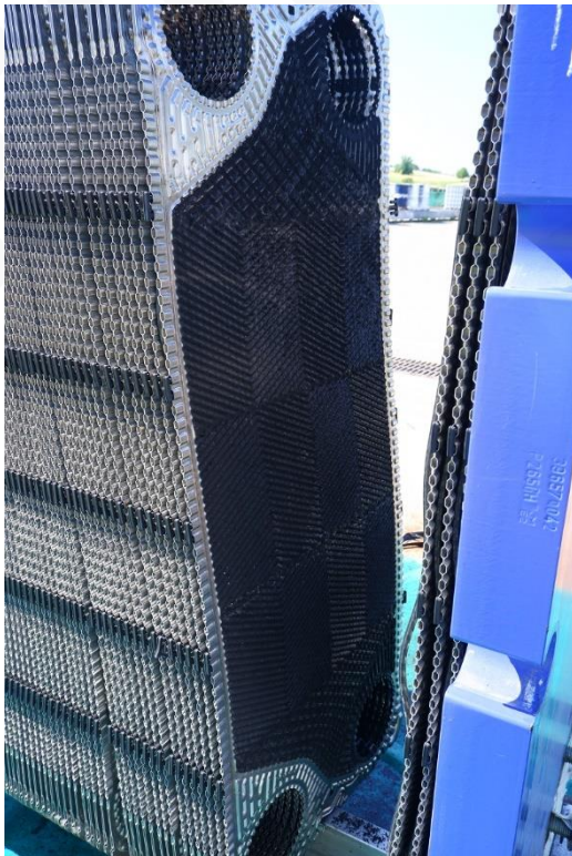
Dismantling of heat exchanger.
