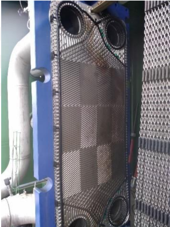
Dismantling of heat exchanger.
